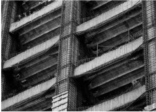
Fig. 3. Concrete jacketing of columns and beams [8]
