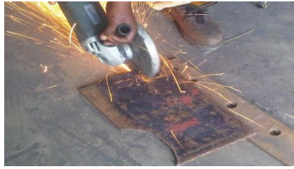
Fig. 4(a). Cutting the Top Plate for the Casing
