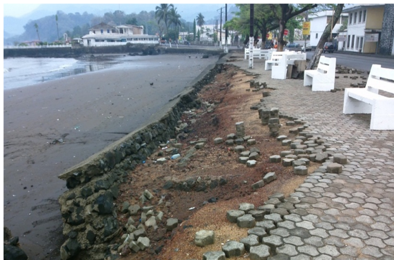
Figure 3. Sea Level Rise and Coastal Erosion of Built-Up Recreational Terraces in Down Beach Coastal Neighbourhood, Limbe
